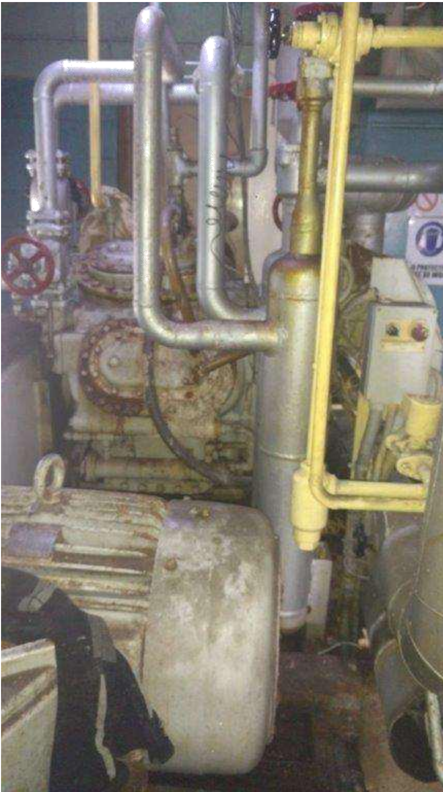
Pafco ammonia compressor repair
